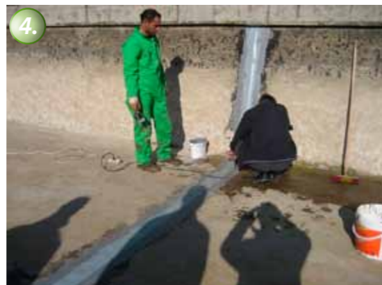
4. Connections are made with a hot air welding gun; seams should overlap at least 2 cm.
