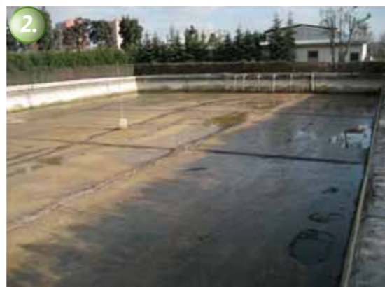
2. The surface is cleaned down to a solid and stable base material. The substrate must be clean, solid, and free from adhesion inhibiting materials.
