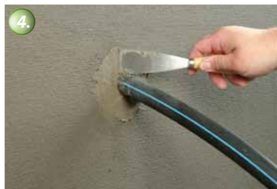
The pipe penetration is now permanently waterproofed.
