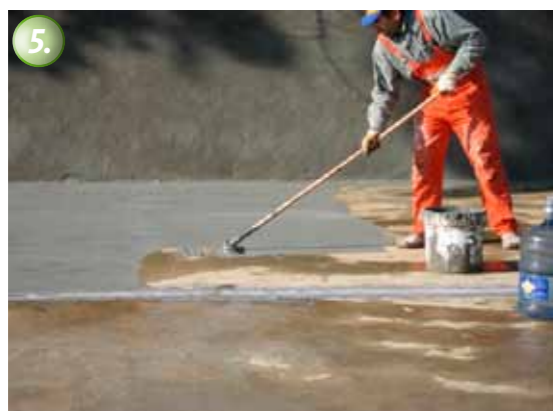
5. The area waterproofing is done with KÖSTER NB 1 Grey. KÖSTER NB 1 Grey is a mineral based waterproofing against ground moisture, non-pressurized and pressurized water. KÖSTER NB 1 Grey is resistant to positive and negative side water pressure.
