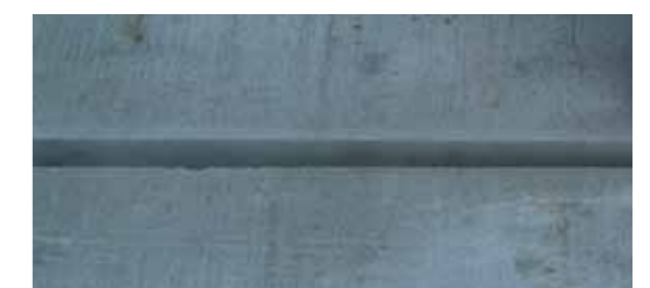
Cleaned joint flanks
