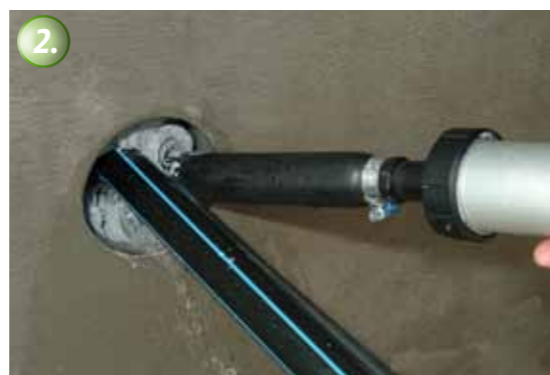
The material is pressed into place between the cable and the wall with the KÖSTER Special Caulking Gun, immediately and permanently stopping the water flow.
