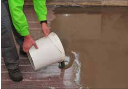
4 Distribute the material in the desired layer thickness directly after mixing (min. three minutes)
