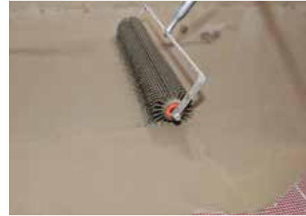
6 Lastly a KÖSTER Spiked Roller is used for de-airing
