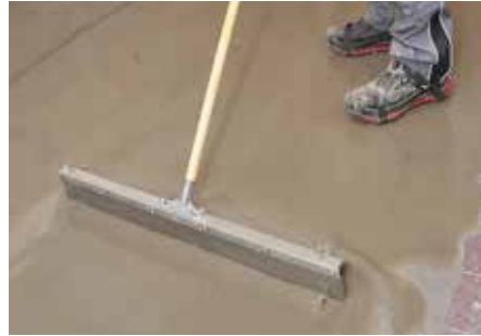
5 When working larger areas use a KÖSTER Gauging Rake to distribute the material
