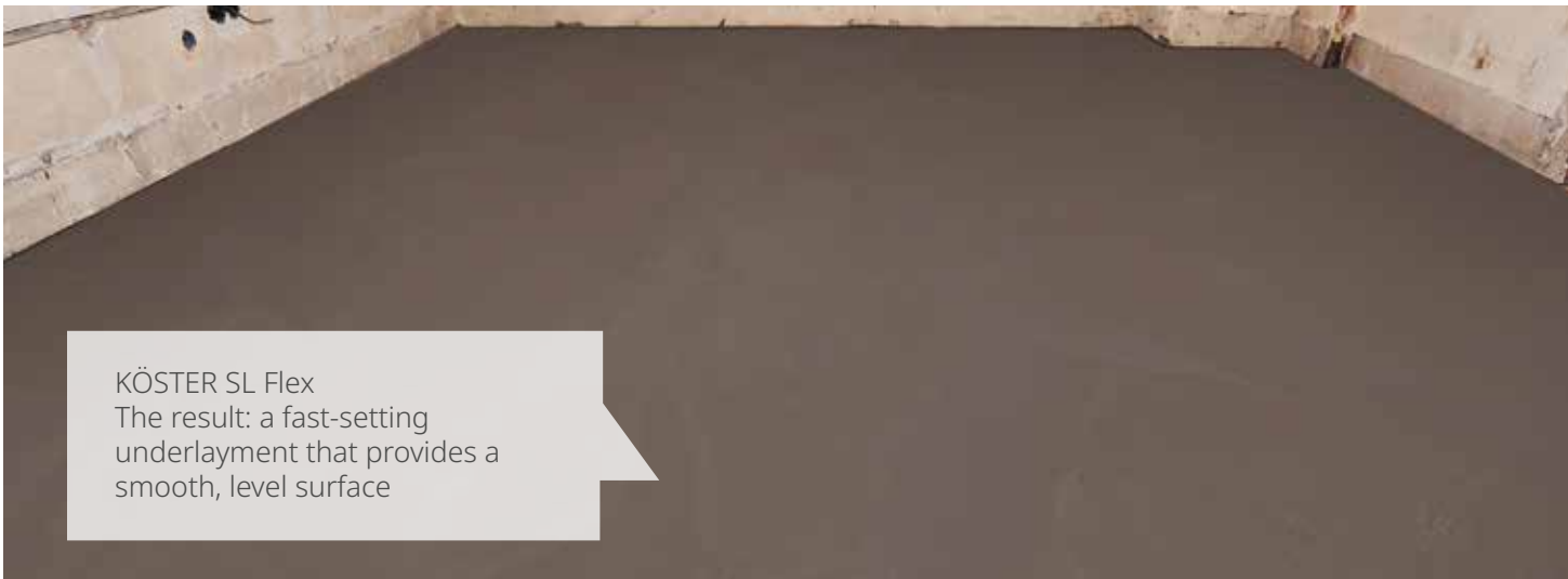
4 Distribute the material in the desired layer thickness directly after mixing (min. three minutes)
